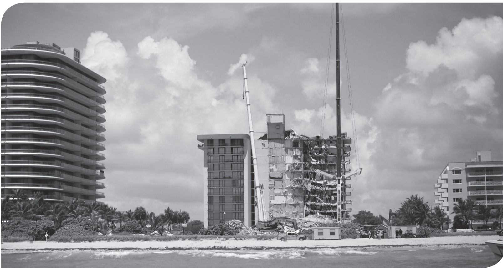
OPERASI PENYELAMATAN KORBAN GEDUNG ROBOH DI FLORIDA - AS
